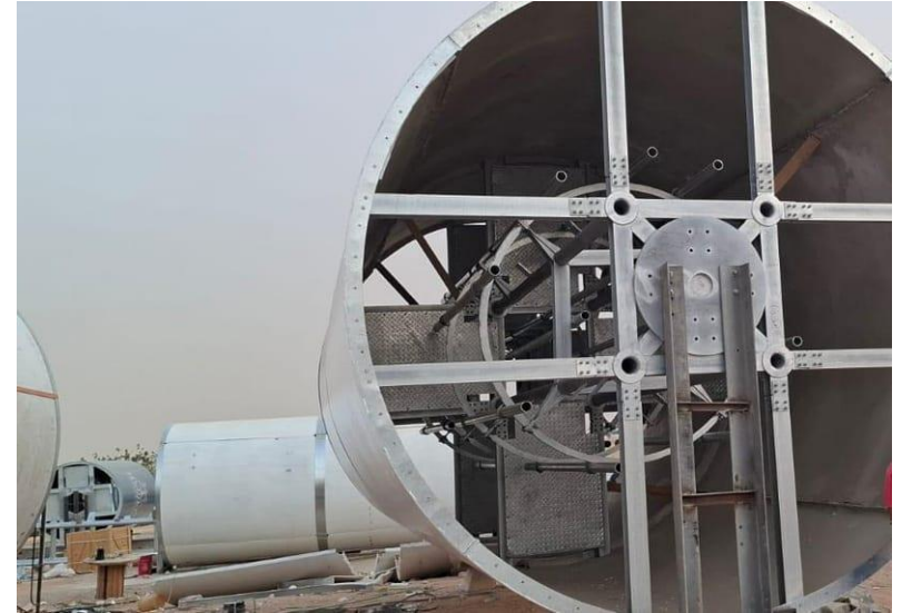
Internal ring framing and central connection hub.
