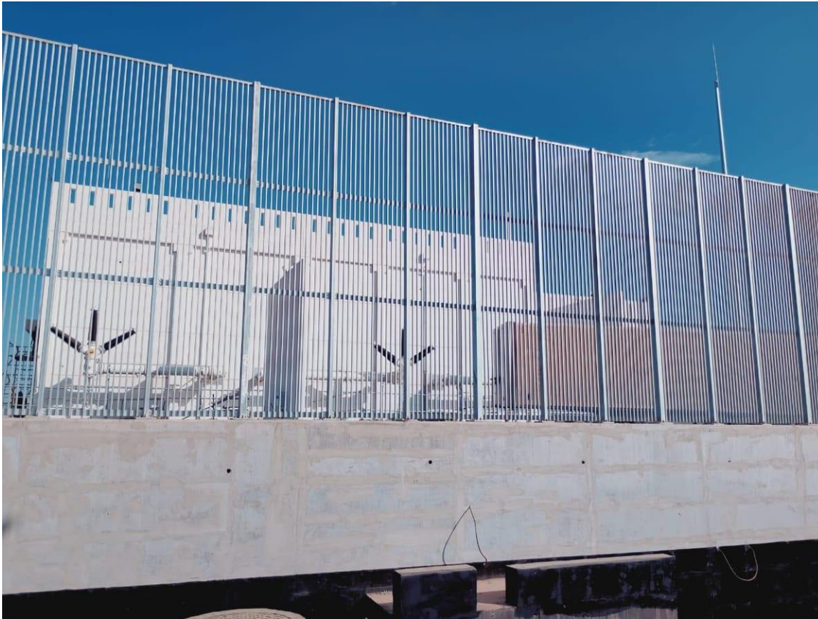
Vertical-bar steel screen fence above a concrete wall.
