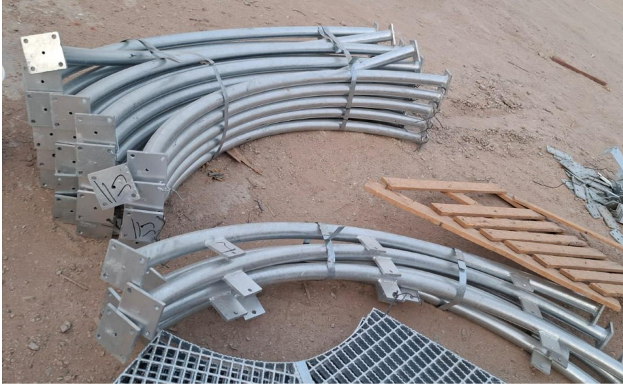
Tubular column with flanged base plate and gusset stiffeners during fabrication.
