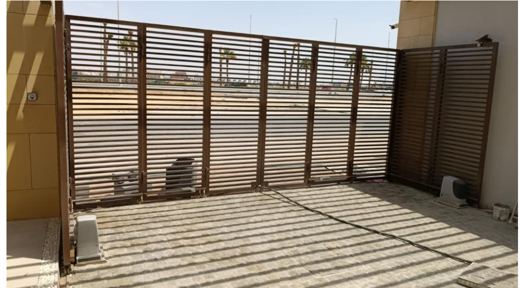
Gateway during erection.
