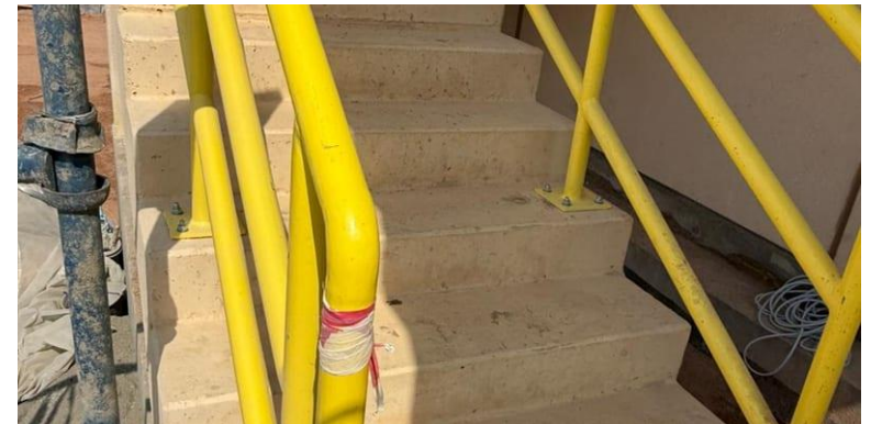
Tubular stair handrail with base plates.
