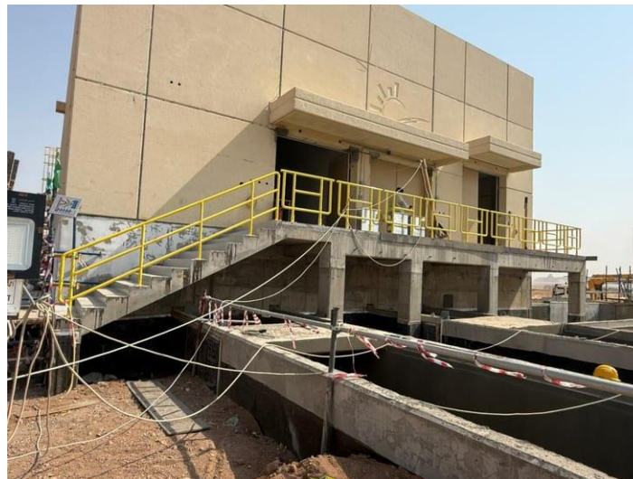
Painted stair and handrails at an elevated entrance platform.
