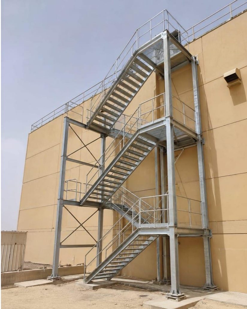
Galvanized three-flight stair tower with landings and handrails.
